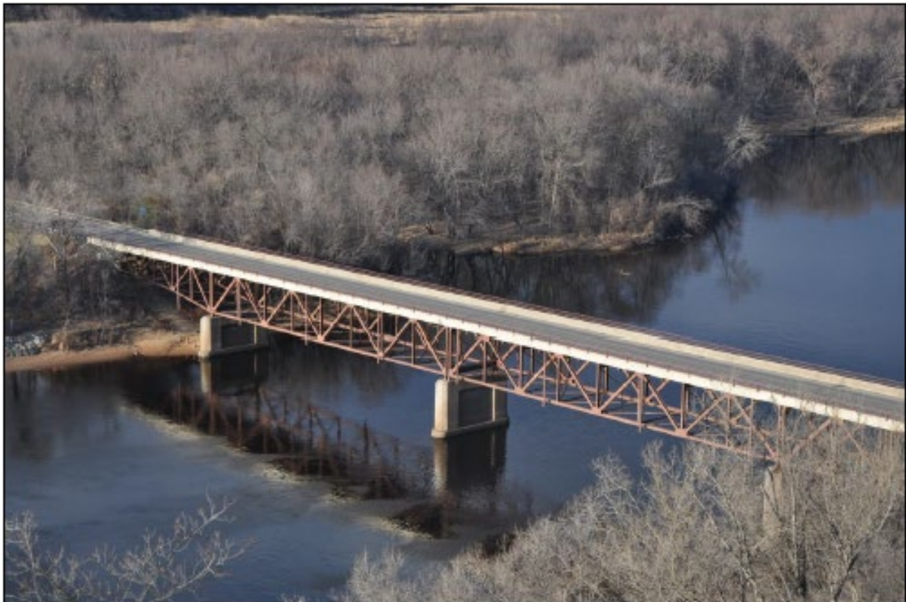
Figure 2-1. Hwy 243 Bridge Over the St. Croix River
