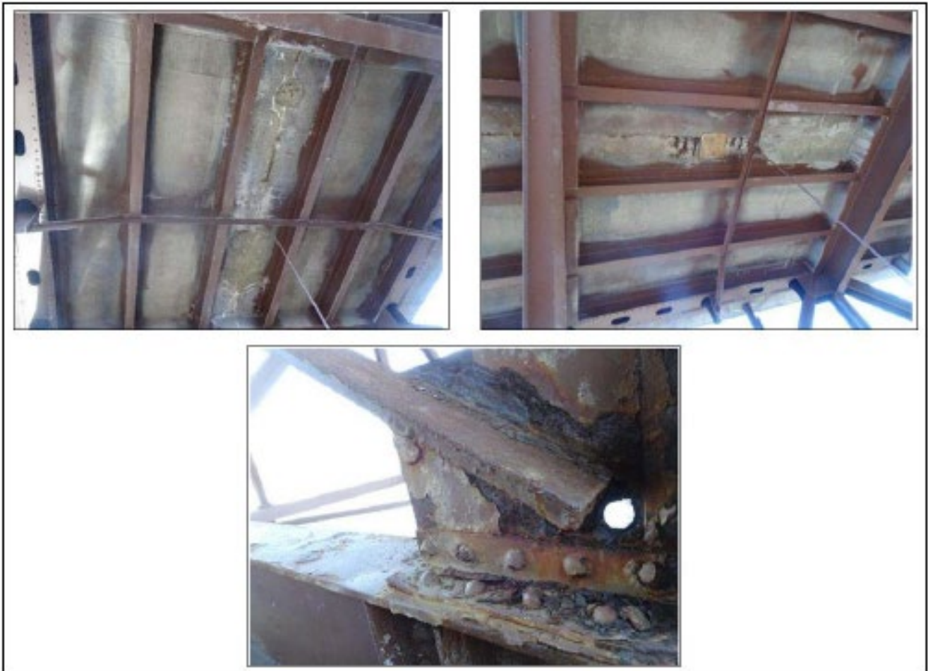
Figure 2-2. Underside of Hwy 243 Bridge Deck and Steel Truss
